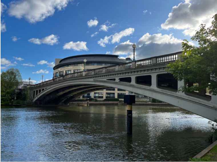
Bridge from the south west (Helen Lambert)
